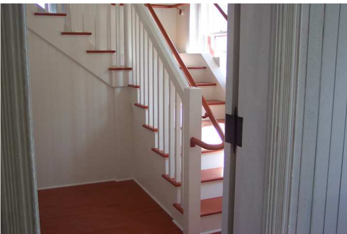
New staircase to 2nd floor, painted
