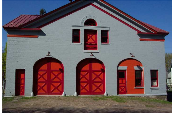
Front view of Carriage House Theatre
